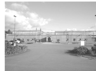
Southern State Correctional Facility Springfield, VT [Photo by Vermont Dept. of Buildings & General Services]
